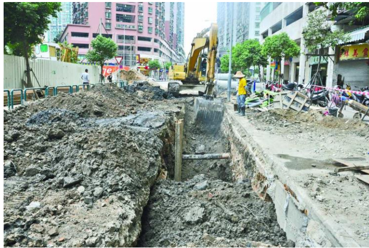
Figure 8 Drainage system is upgraded in old districts.
